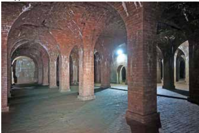
Papplewick Reservoir: the brick columns and vaulted roof. The view shows about half of the reservoir. Photo Clive Penfold
